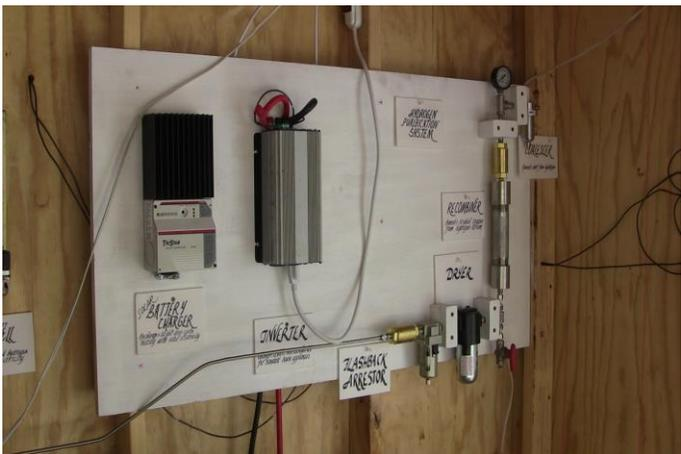
PV electronics and H2 purification system
