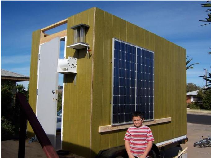
Solar panels, electrolyzer & Bubbler in place
